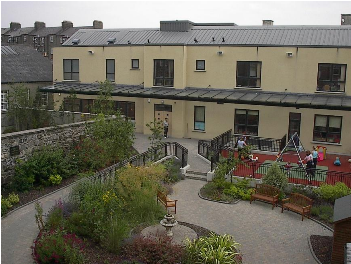
Garden, Nursery & CTC Building
